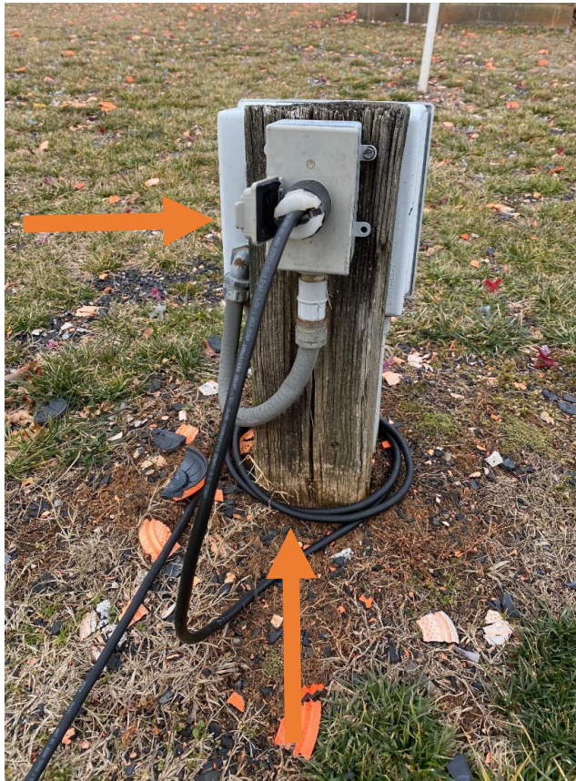
Best practice includes wrapping cord around receptacle post a couple times before plugging in
